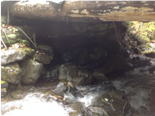
Left Bank Abutment when facing downstream
