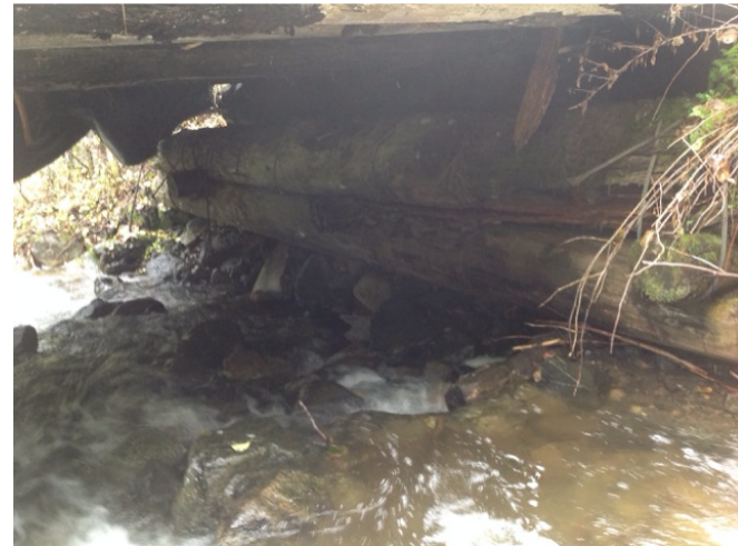
Right Bank Abutment when facing downstream
